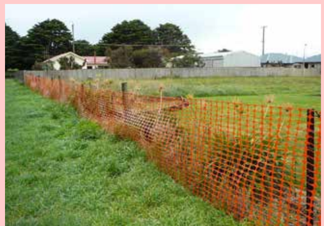
Unsafe scenario where no or minimal perimeter fencing is provided
