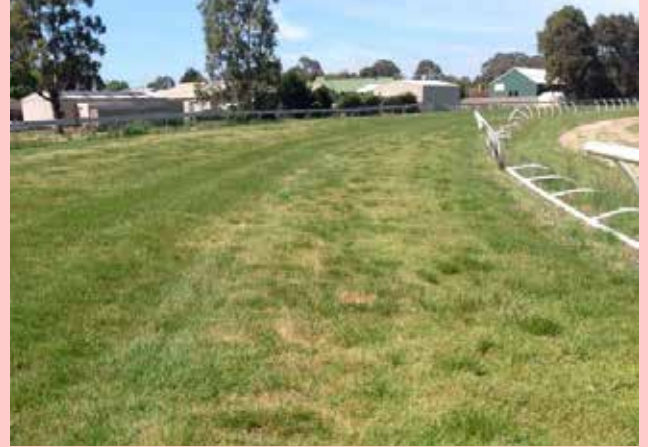
Rails not repaired following an event
