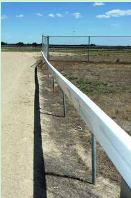
Well-maintained metal rail
