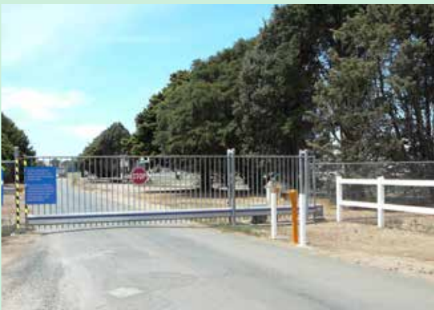
Self-opening gates that are code access for after-hours
