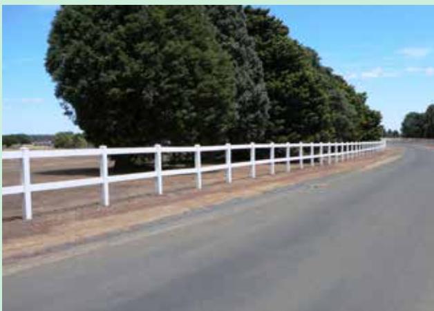
High edge fencing along roads
